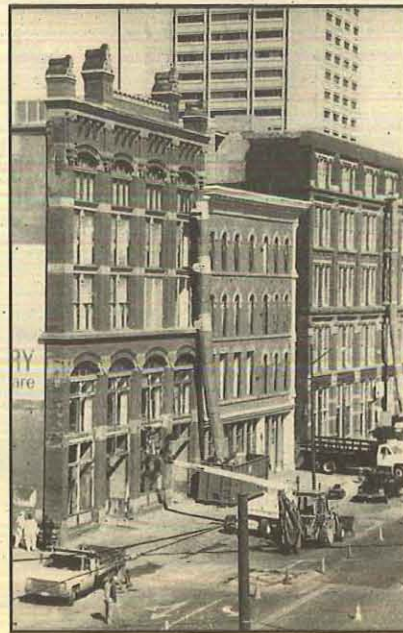
Preservation at work: Rehabilitating buildings in the Warehouse District
